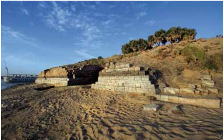
1 Quay walls of Nag el-Tawil at the west bank of the Nile
