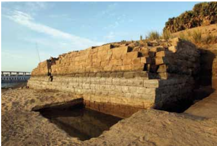
3 Southern jetty of the quay walls
